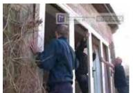
Once in the correct position and the door is plumb and square without twist, you can begin fixing the door into the opening, using appropriate fixings (not supplied). When fixing down to the cill, ensure that screws are sealed to prevent water ingress. Also seal across the cill below the door jambs to prevent water tracking across the cill.
