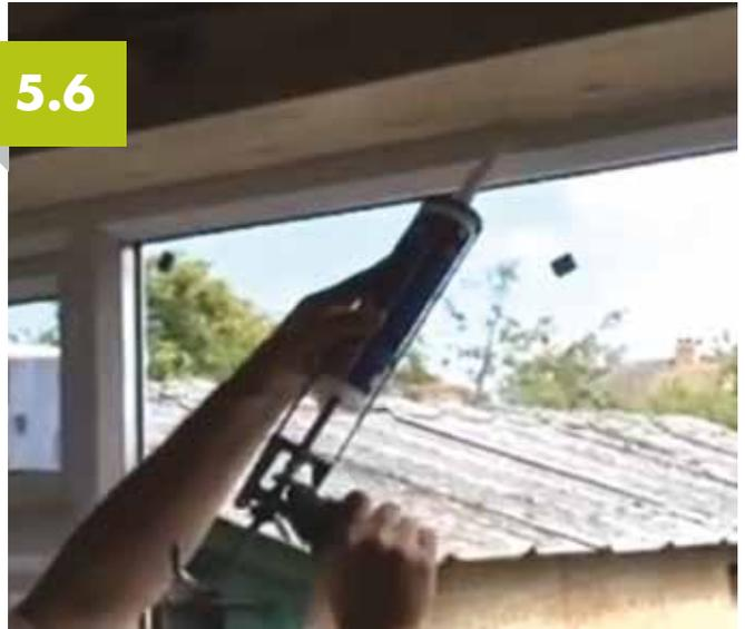
Run a strip of masking tape around the frame, then apply a bead of sealant between the frame and the wall. Remove the tape before the sealant sets. Apply this step to all four sides of the frame.
