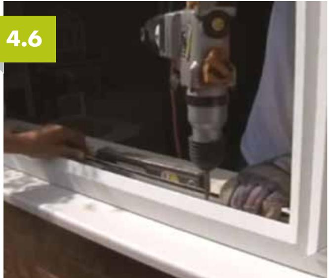
On wider frames don't forget to fix the top and bottom of the frames, this will help prevent deflection in windy conditions. Ensure that any holes drilled in the bottom of the frame are sealed with silicone to prevent moisture absorbing into the brickwork.
