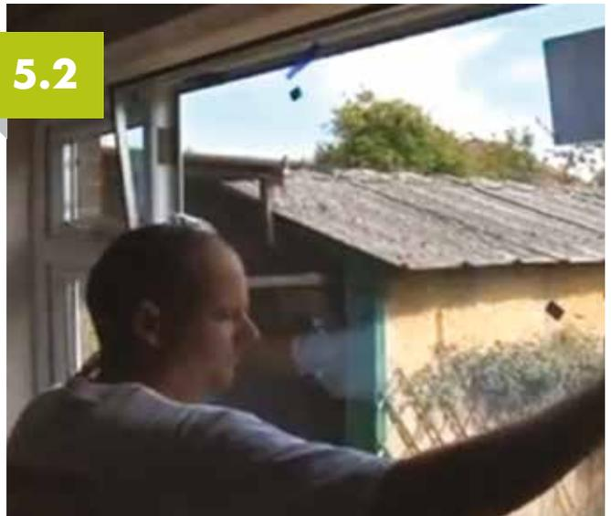
Place each pane into position, noting that where opening casements are hinged from the sides they should have the glass packed at diagonally opposing corners to hold the casement square.
