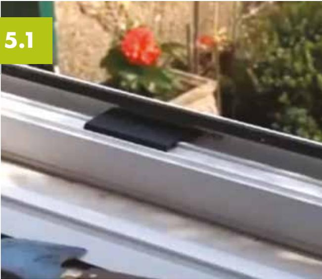
Commence glazing the frame, ensuring that appropriate glazing platforms are fitted around each aperture. These centralise the glass and allow free passage of water to run to the drainage slots.
