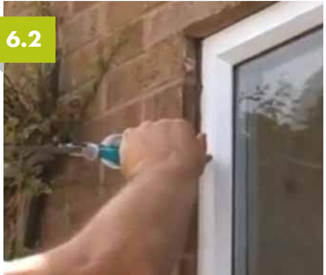
Apply a strip of masking tape to the frame perimeter. Apply a smooth bead of silicone sealant between the frame and brick work. Before the sealant sets, remove the making tape to create a neat finish.
