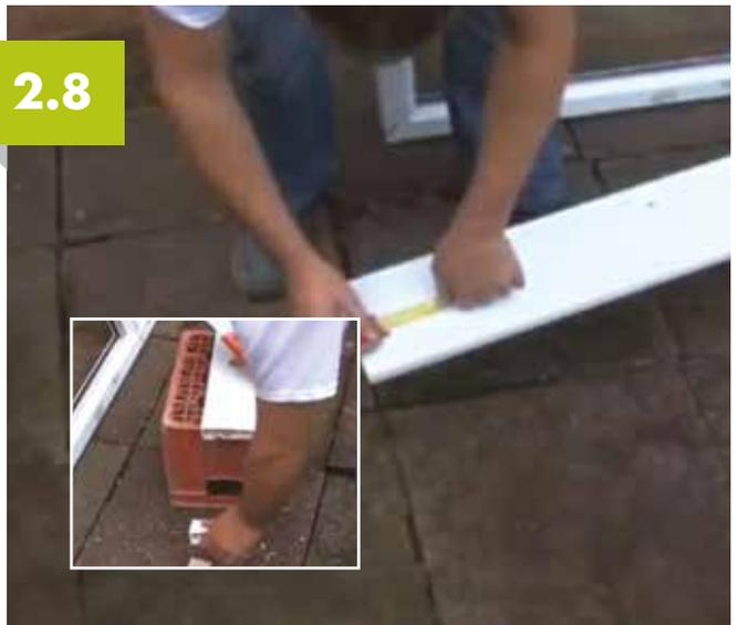
Prepare the external cill for fitting to the new frame. This can be done one of two ways, either fitted full width or rebated around the brickwork to achieve a neat finish.
