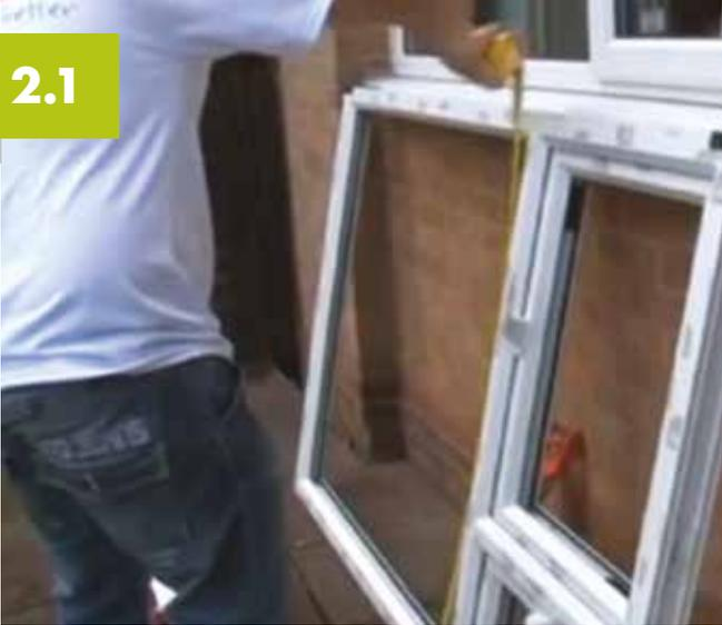
On arrival, before removing any existing window frames, check that the replacement frames size is the same as the existing window frames. When checking the sizes, ensure that the new frame has a 5mm expansion gap around the perimeter.
