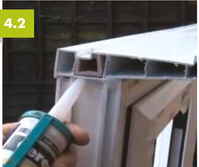
Be sure to seal the ends of cill and frame assembly to prevent moisture from tracking along the cill and into the brickwork.
