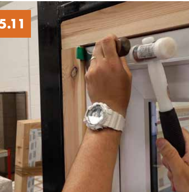
Cut off the packers flush to the frame.
