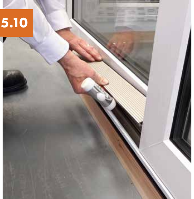
Position the cill cover/low threshold cover.
